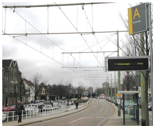
Figure 6-3 ITS for Public Transport: Information about the Next Arrival at the Tram Stop
