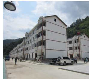
8 resettlement centralized sites were constructed
